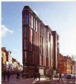
1. Sauerbruch Hutton's BSU Office for Urban Development and the Environment in Hamburg displays a bold use of colour 2. DSDHA's 28 South Molton Street, London store for Bosideng is a striking bespoke terracotta building
